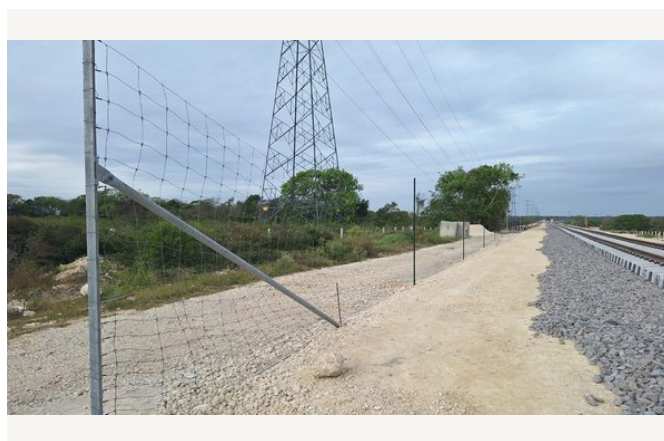
Perimeter enclosure alongside the railway.
